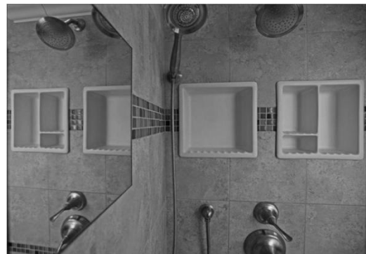
Figure 3. Grout around the mirror to seal and finish.
