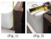
measure where to install the support frame. (Fig.1) Shimming may be necessary to move the sink up to the solid surface or to make the sink drain properly. A reveal of 1" to 2" inches is common. (Fig. 2)
