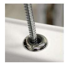
Water from the hose can drip down into the hand shower base and get behind your tub without the barrel protection.
