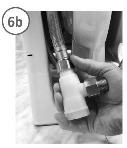
7a. Hand-tighten 1/2" supply line (included) to the 1/2" brass filter adapter.
