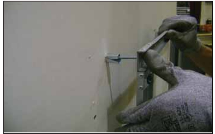
Figure 4.6 Installing Anchors in Hollow Wall
