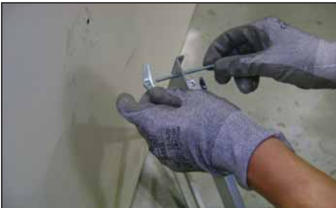
Figure 4.5 Toggle Bolt Installation through Mounting Bracket
