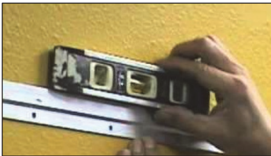
Figure 2. Locating position of Z-bar bracket.
